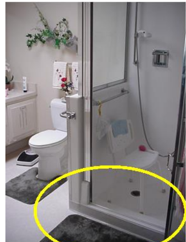
After Cut Down
